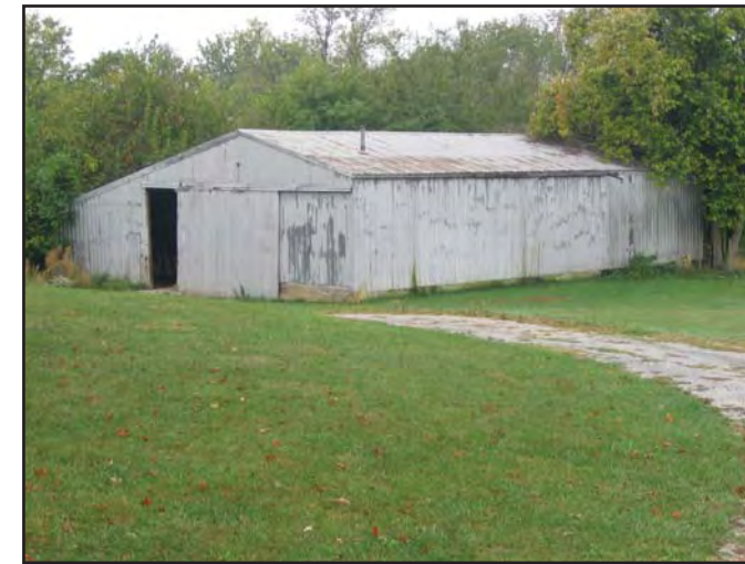
View of Maintenance Shed
