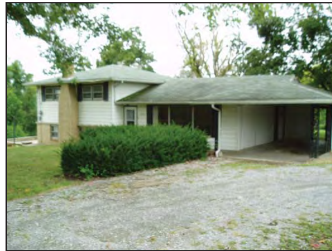
Front view of Existing Residence
