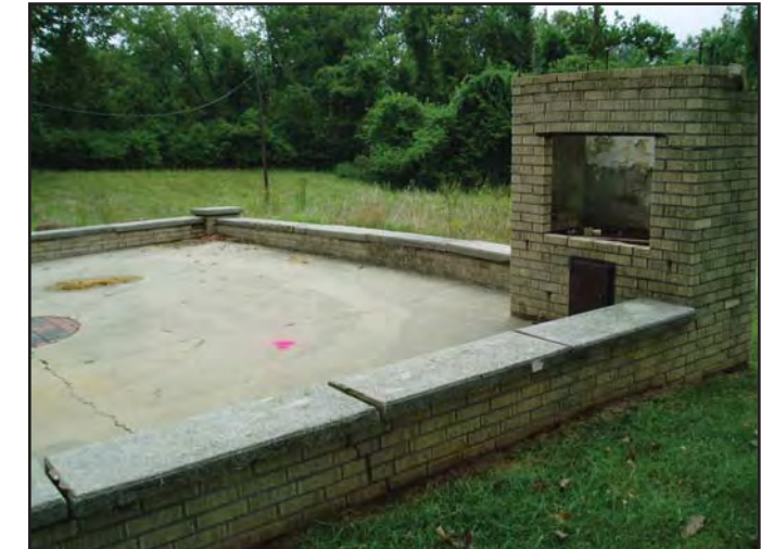
View of Existing Patio at South Side of Residence
